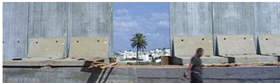
ΝΟΤΟΣ/SOUTH – CAS 13/3 13:00, ΚΕΝΤΡΟ/CENTER – ZAN 11/3 11:00 - MAR 13/3 20:30 ΒΟΡΡΑΣ/NORTH – ZAN 12/3 11:00 - CAS 14/3 20:00 #47 ●
